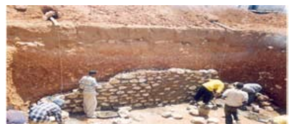
Plate 7: Construction of underground cistern for harvesting rain water in Deri-mara village
