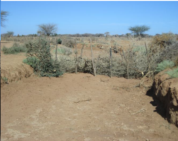
Rehabilitation of an irrigation Canal in Galoolay village and lining vegetation barriers to heal gullies. (Photos are from a project funded by Save the Children Alliance)
