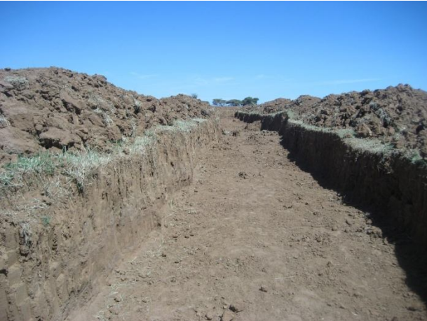
Rehabilitation of an irrigation Canal in Galoolay village and lining vegetation barriers to heal gullies. (Photos are from a project funded by Save the Children Alliance)
